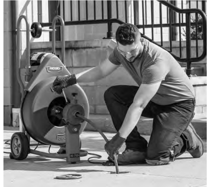
Figure 14 – Operating the K-750 using the AUTOFEED
